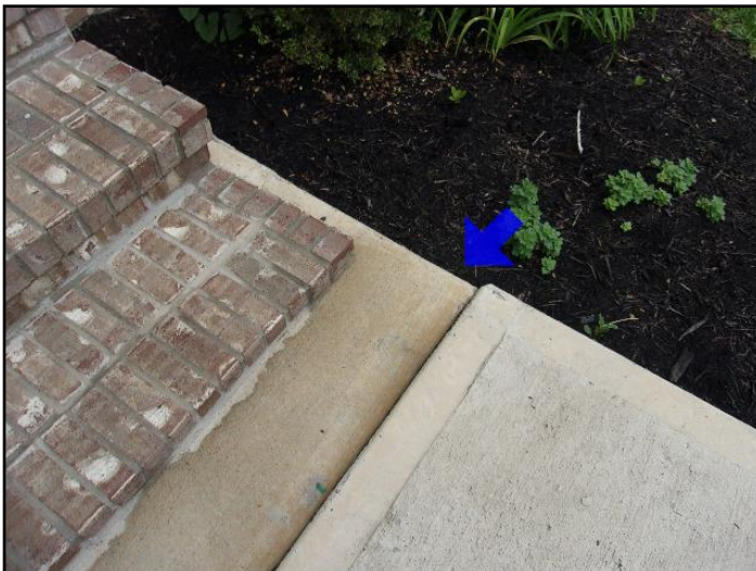
2. Steps or landings settling or heaving
