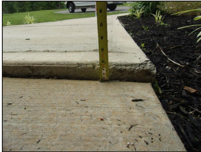
4. Steps or landings settling or heaving
