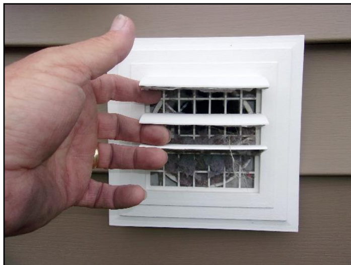
10. Dryer vent obstructed
